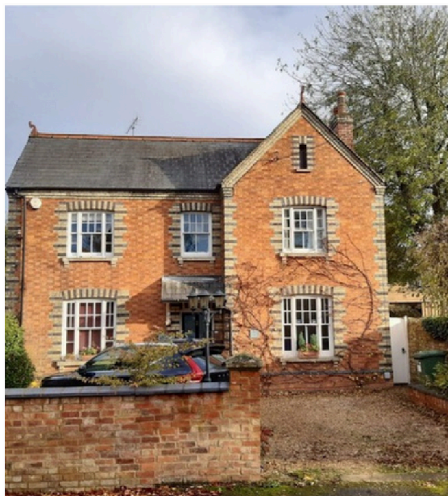
The School and School House are notable for the use of 'polychrome' brickwork.
