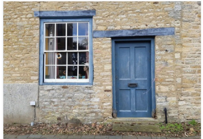
Window and door at 3 High Street.
